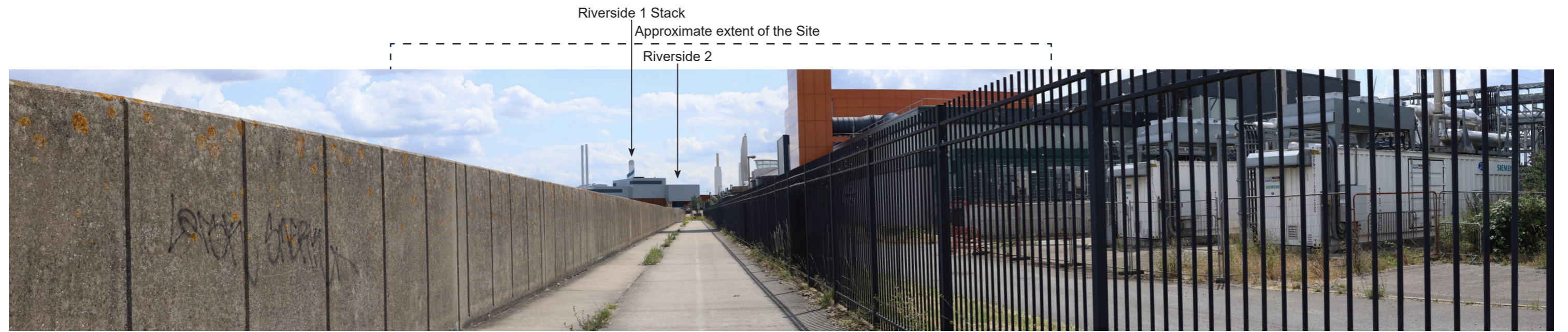
Sequential View 2: From England Coast Path, National Cycle Network Route 1, and Public Right of Way FP2, looking east
